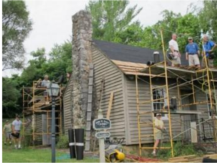
Volunteers roof the Early Cabin in Fincastle
